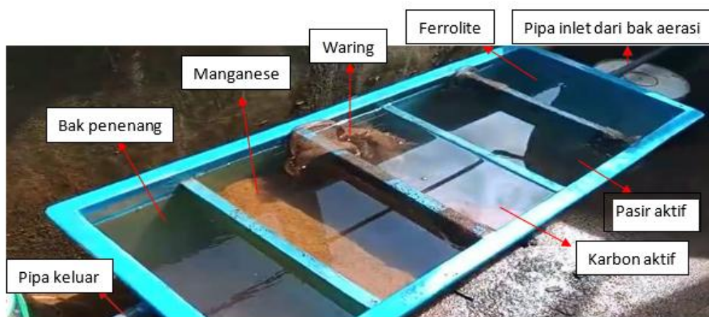
Gambar 4. Susunan Media Filter
